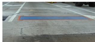
In-motion Road Weigh Bridge
